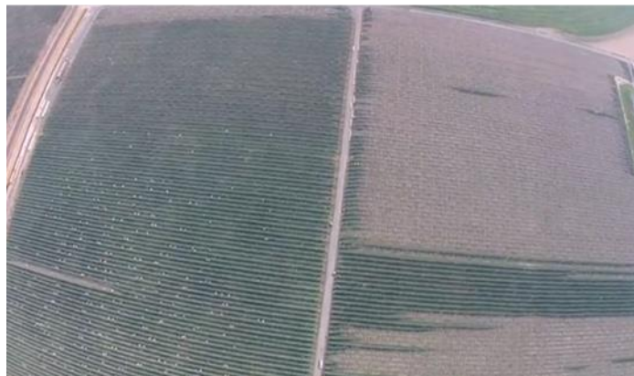
Figure 6. Aerial view of failed trellis (right) with end posts still standing.
